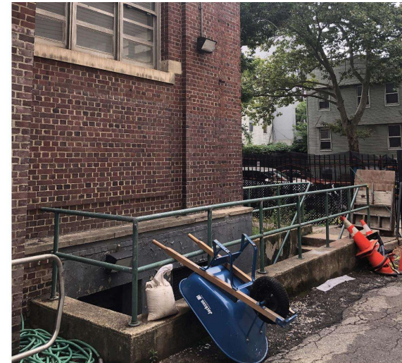
PHOTO 8: EXISTING VIEW OF EAST ELEVATION - EXISTING STAIRS FROM BOILER ROOM
